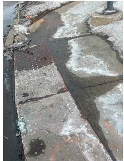
Figure 14: Sidewalk Condition at 15 Mile and Van Dyke. Shows weathering near curb ramps.
